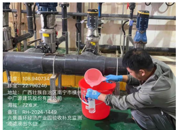
渗滤液进口采样
